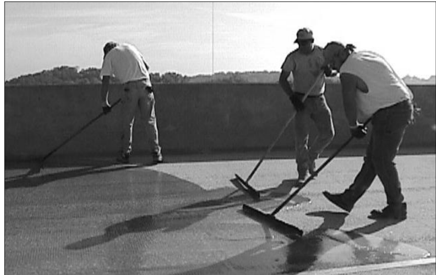
The first coat of polymer is applied with a notched squeegee.
