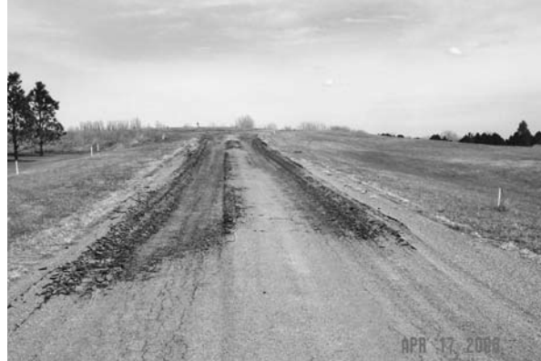
These photos show the difference between an extremely thin base on very weak subgrade soil (top left) and a deep, good quality base gravel on a very sound subgrade (bottom left). The road above, in South Dakota, failed after just one year because of a very poor base. You cannot break basic rules of planning, designing and construction of roads and get long-term performance.
