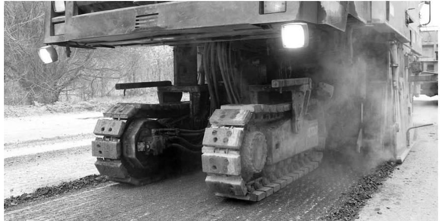
The quality of reclaimed asphalt pavement (RAP) is dependent on the age and quality of the asphalt from which it is derived. RAP can be amended to improve its performance.
